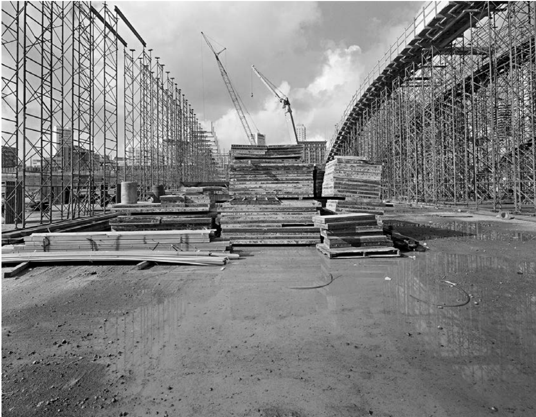
Arch Construction II, George Moscone Site, 1981
